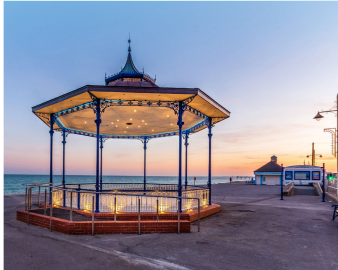
Bandstand Bognor Regis seafront, council received £50k Coastal Revival Fund grant towards its renovation
